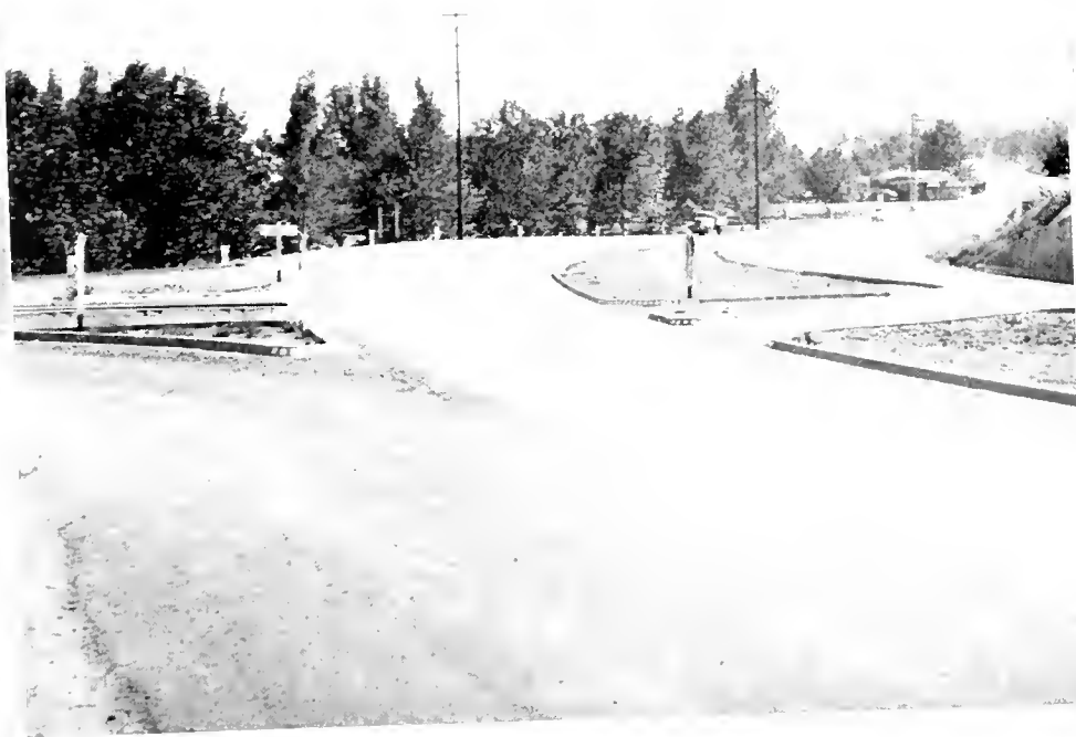
Views of channelization project recently completed on U. S. 99 near Redding that converted the existing 2-lane road into a 4-lane divided highway. At the 3-way intersection with Route 20 and the highway to Volcanic National Park, opposing traffic is separated by irregular shaped division strip areas partially bounded by concrete curbs.
